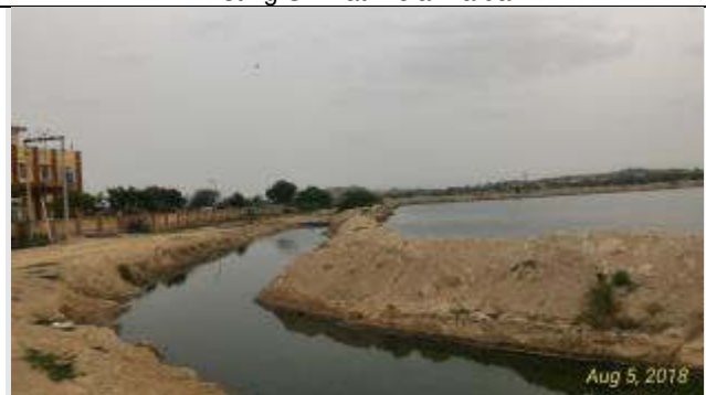
Effluent discharge of existing STP in lagoon
