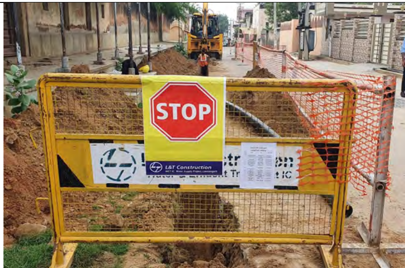
Pipe laying works in small sections
