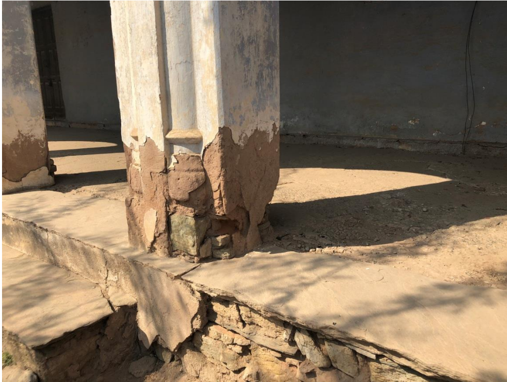
Source 13 Author Figure 35 showing moisture damage at Jai Niwas
