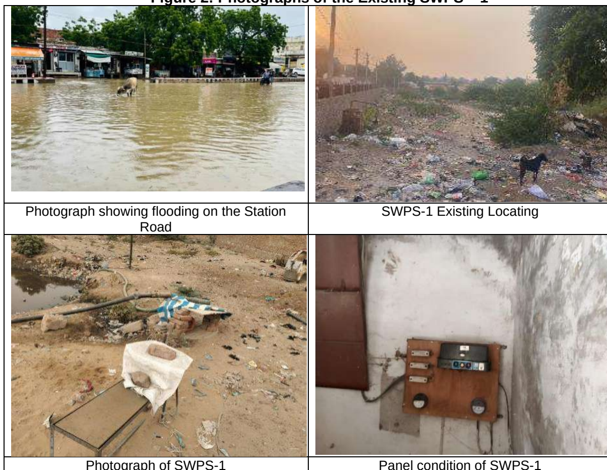
Figure 2: Photographs of the Existing SWPS – 1
