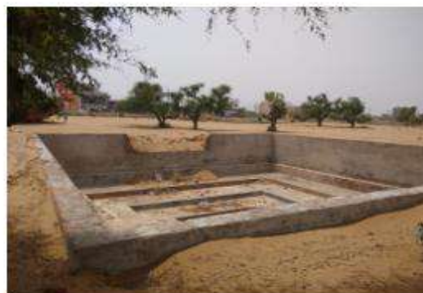
Chainage- 1850 BADRANA JOHAD Disposal point
