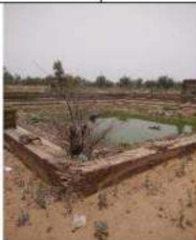
CHAINAGE 200 - Disposal point at BAWADI
