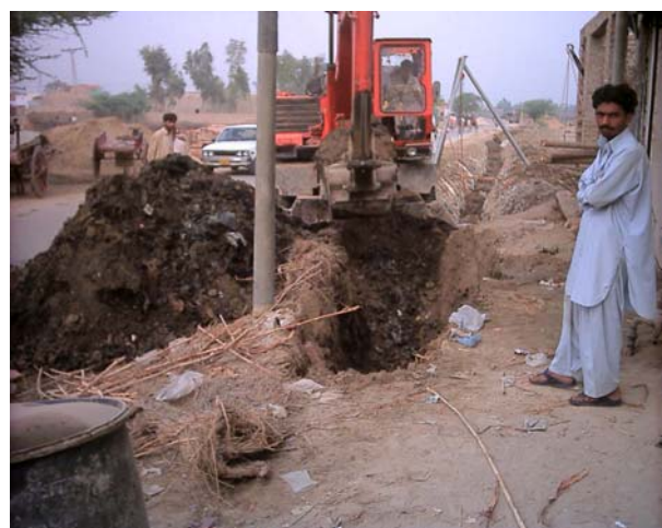
Photo 30: Backhoe digger for trenching
