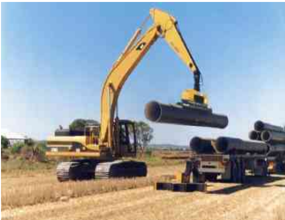
Photo 32: Crane for laying pipes
