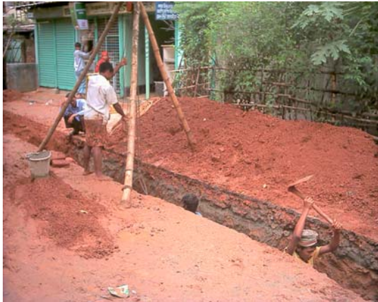
Photo 31: Digging a trench by hand
