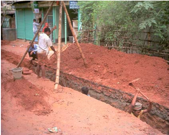
Photo 18: Digging a trench by hand
