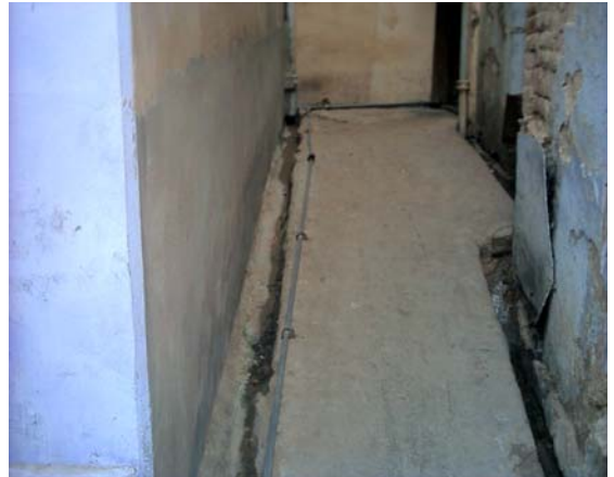
Photo 21a: water supply pipe above ground
