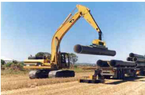
Photo 19: lying of pipeline using crane
