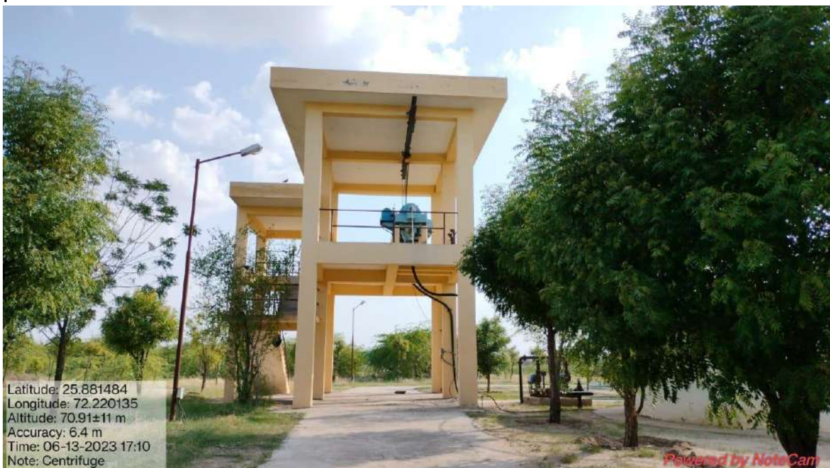
Temporary RCC structure with centrifugal pump, for dewatering and Sludge drying
