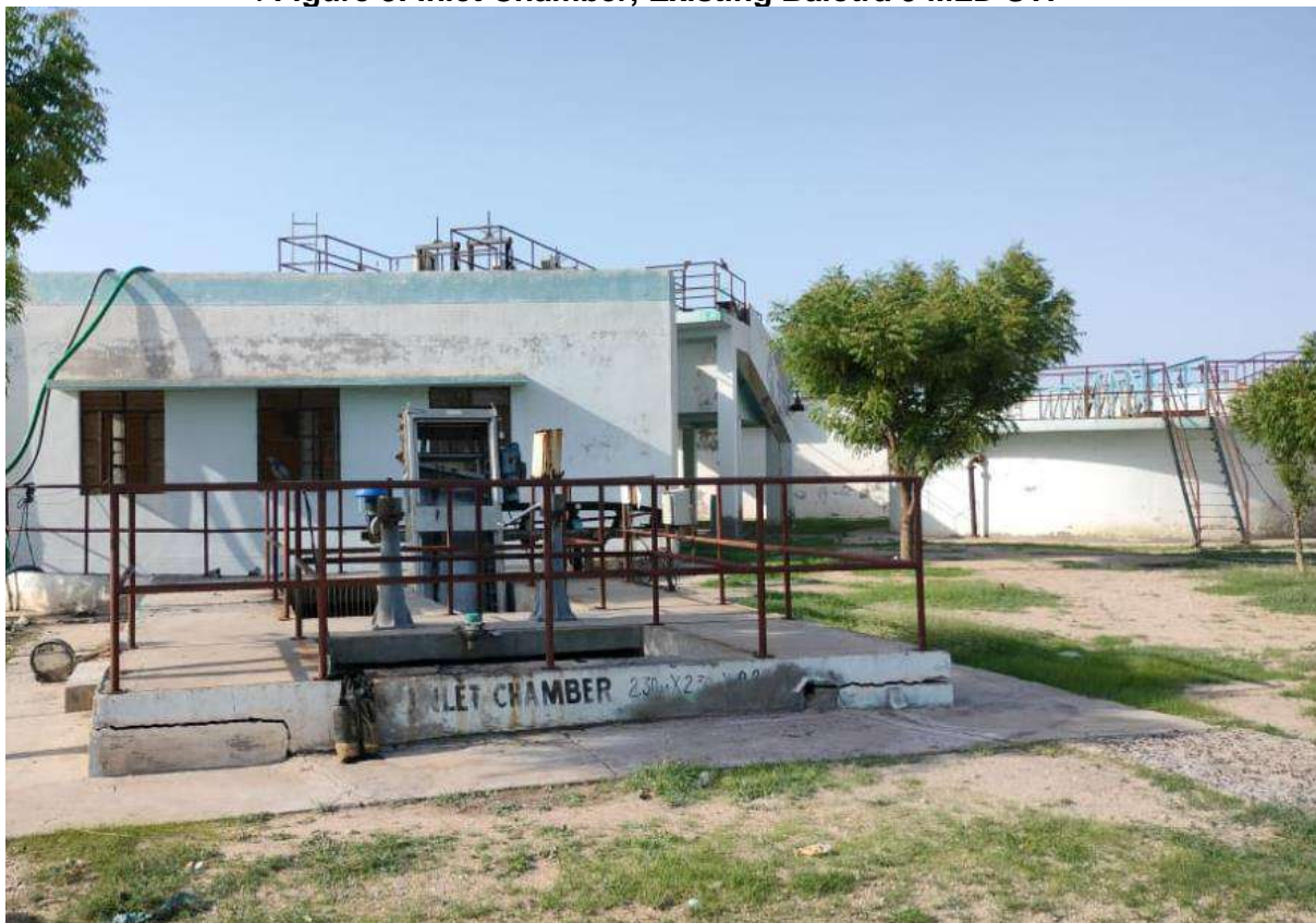
. Figure 3: Inlet Chamber, Existing Balotra 9 MLD STP
